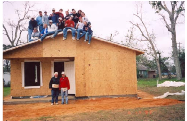
One of the houses, ready for the first inspection.
