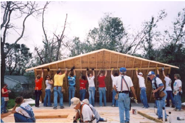
Starting with a slab of concrete, the walls go up...
